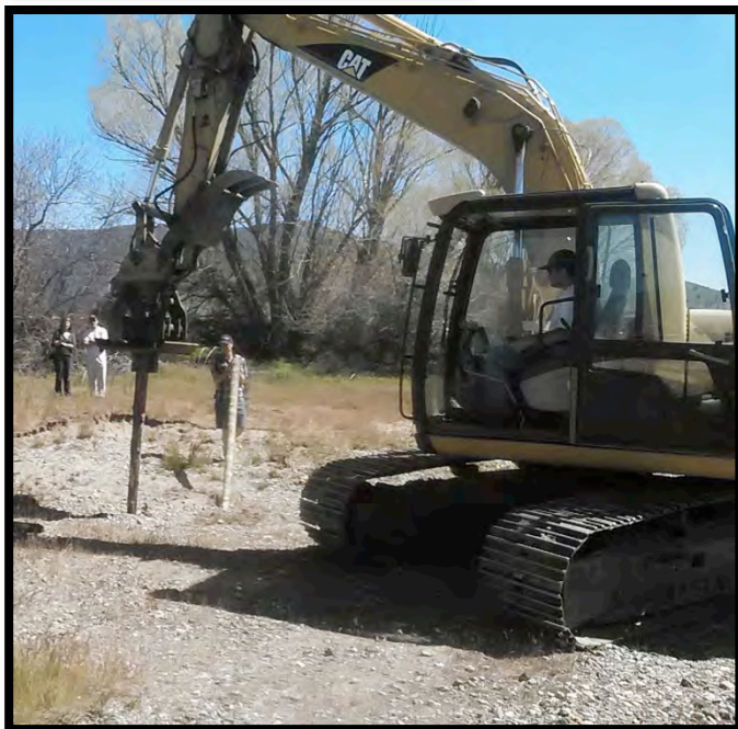
Figure 27: Hydraulic post pounder options. Options include, clockwise, starting from upper left: (a) a hand-held pounder attached to hydraulic power pack, (b) a post pounder attached to bulldozers, (c) a handheld pneumatic post pounder attached to an excavator and (d) a modified excavator with a vibrating pad. Options (a) and (b) take approximately 5 to 10 minutes per post, depending on substrate, and it can be difficult to get to the desired depth. Option (d) takes less than 1 minute per post and can drive posts as deep as needed. All pounders have a metal cylindrical cap that holds the post in place while pounding. Each option has pros and cons to consider, including cost, maximum depth the posts can be pounded, substrate type, operator strength and expertise, and the amount of likely riparian and instream disturbance. Photo credits: (a) Nick Weber, Ecological Research, (b) Mark Cookson, USFWS, (c) Peter Thamer, Siskiyou County Resource Conservation District, and (d) Julie Ashmore, Okanogan Highlands Alliance.
