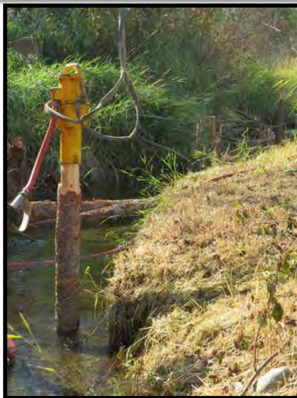
Figure 27: Hydraulic post pounder options. Options include, clockwise, starting from upper left: (a) a hand-held pounder attached to hydraulic power pack, (b) a post pounder attached to bulldozers, (c) a handheld pneumatic post pounder attached to an excavator and (d) a modified excavator with a vibrating pad. Options (a) and (b) take approximately 5 to 10 minutes per post, depending on substrate, and it can be difficult to get to the desired depth. Option (d) takes less than 1 minute per post and can drive posts as deep as needed. All pounders have a metal cylindrical cap that holds the post in place while pounding. Each option has pros and cons to consider, including cost, maximum depth the posts can be pounded, substrate type, operator strength and expertise, and the amount of likely riparian and instream disturbance. Photo credits: (a) Nick Weber, Ecological Research, (b) Mark Cookson, USFWS, (c) Peter Thamer, Siskiyou County Resource Conservation District, and (d) Julie Ashmore, Okanogan Highlands Alliance.
